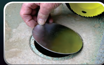
Flush finish, seal with a cavity plate
