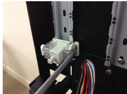
4. Take a flat headed screw driver and insert in to clasp located to the back side of the ECM 1B module. Exert an outward force whilst pushing down the module to engage and lock module into position on the indented din rail.
