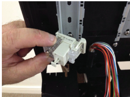
3. Locate and clip the ECM1B screw side on to the indented din rail position.
